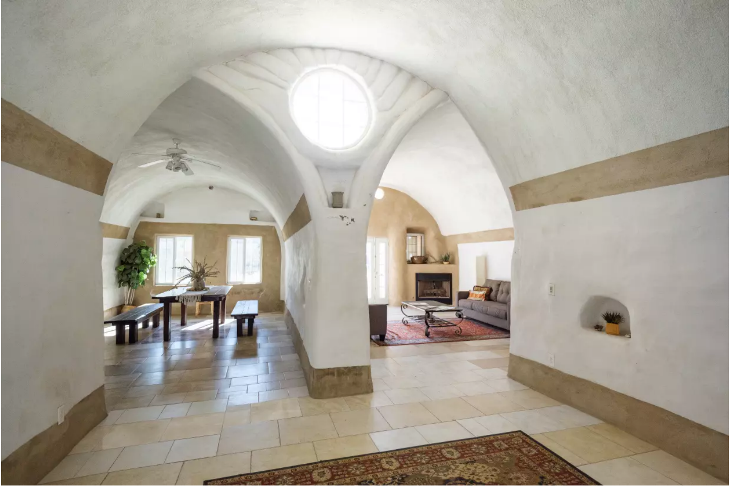
The construction of SuperAdobes relies on the arch, a load-bearing shape. (William Liang / For The Times)
